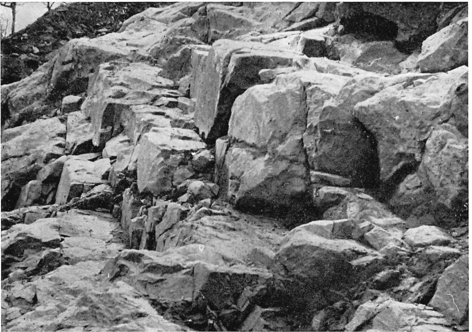
PLATE 2. — Detail of rock structure on right bank with upstream-dipping joints (dipping towards camera).
