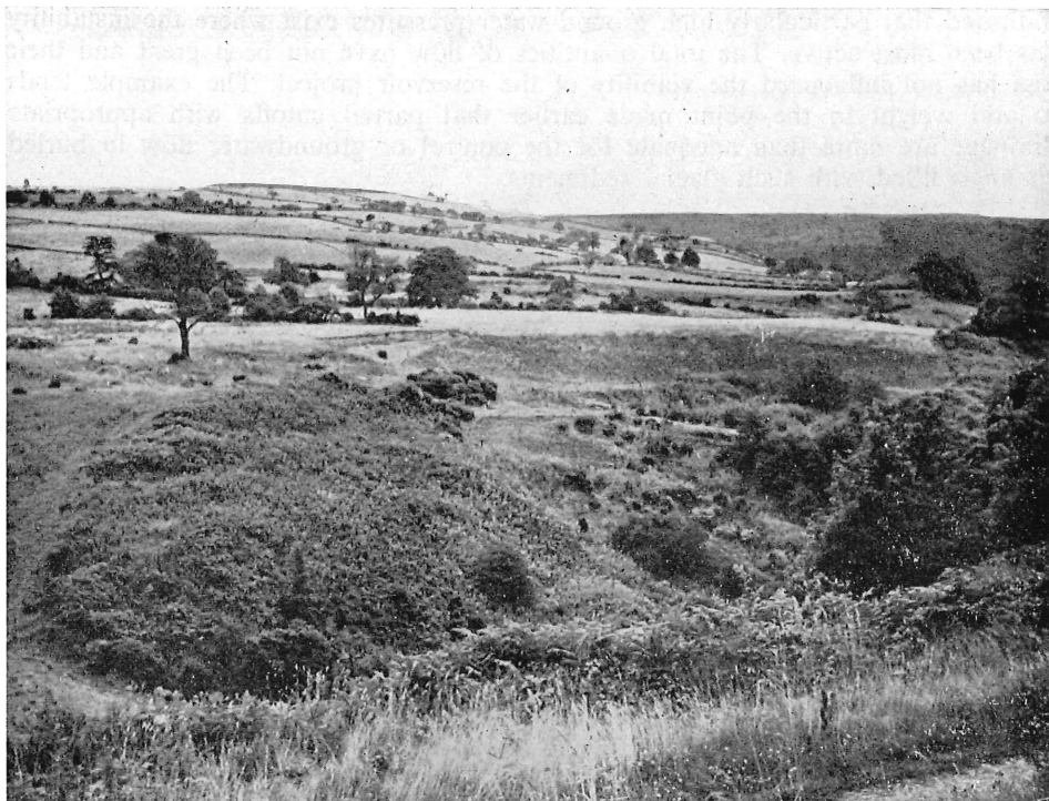
PLATE 8. — View of slips in glacial lake deposits in buried channel immediately downstream of the left bank of the Cod Beck dam.
