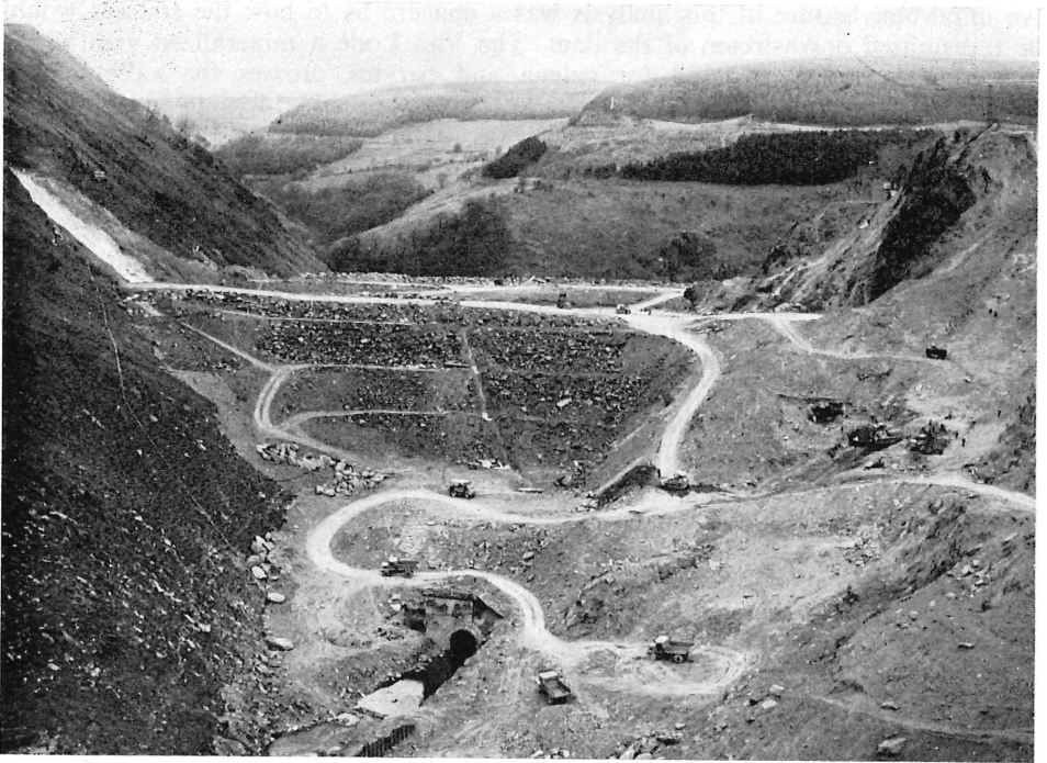
PLATE 4. — General view of Brianne rock fill dam under construction.
