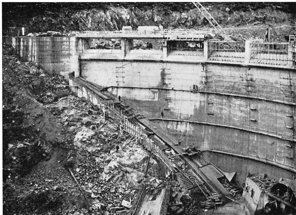
PLATE 1. — General view of right bank of Monar dam during construction.
