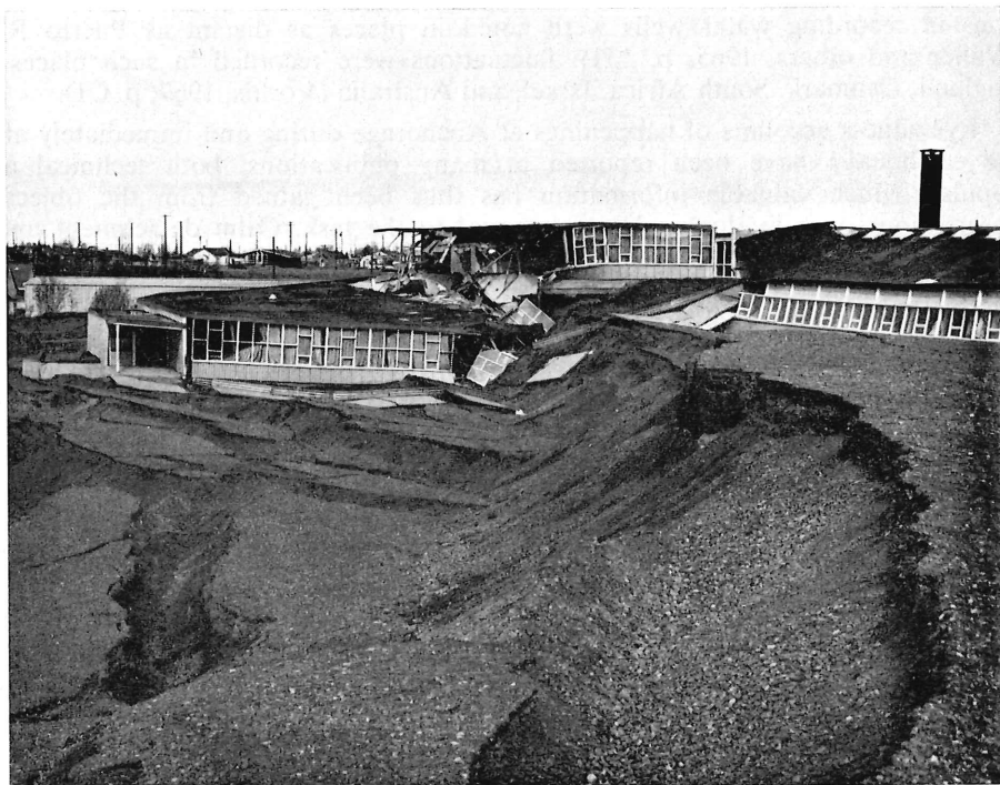
FIG. 2. — Government Hill Elementary School, destroyed by landslide.
