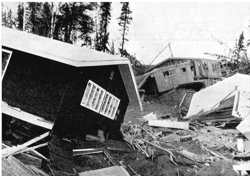
FIG. 10. — Private homes demolished by Turnagain Heights landslide. Seventy-five houses were destroyed in this slide; dozens more were severely damaged.
