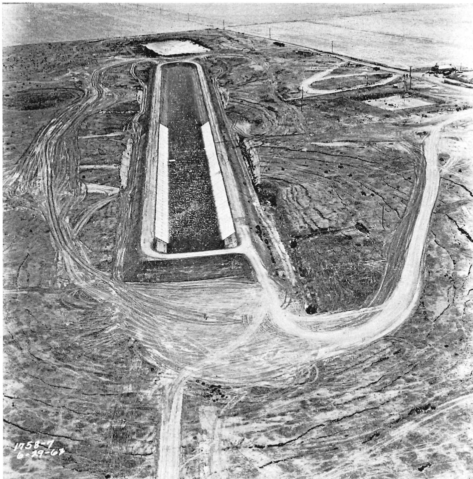
FIG. 9. — Prototype subsidence test. Note peripheral ground cracks due to hydrocompaction.
