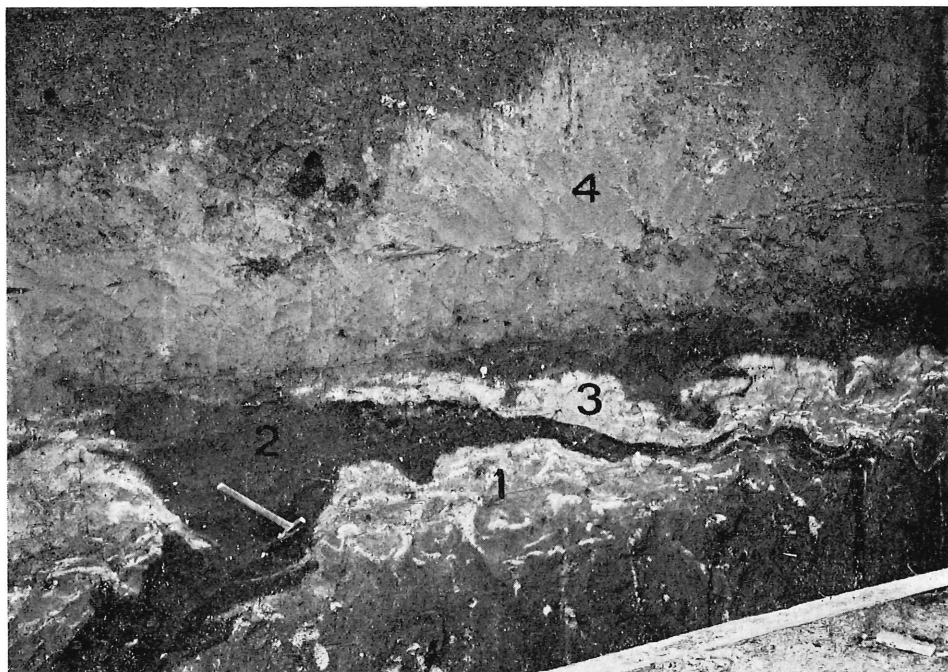
FIG. 6. — Excavation for the foundation of an industrial plant northeast of Prague. 1, weathered Cretaceous marls; 2, frost wedge filled with fossil soil; 3, marls with soil dragged out by soil creep; 4, loess cover. Photo by Záruba.
