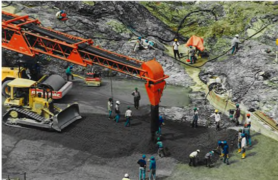
Fig. 1: Handling and spreading of RCC
