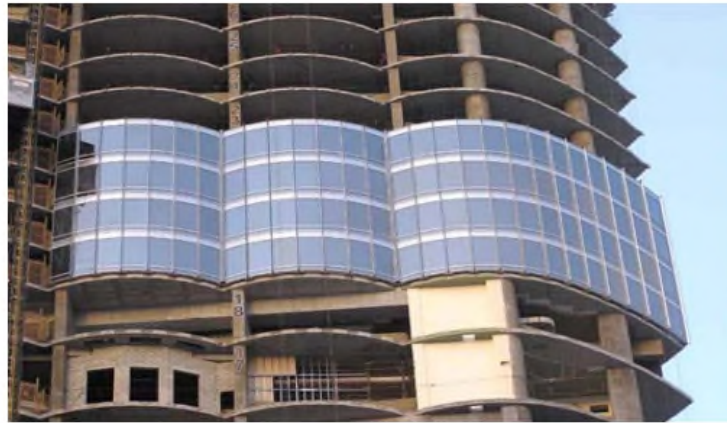
Figure 11: High performance exterior cladding system was used to withstand the extreme temperatures during the summer months in Dubai [9].
