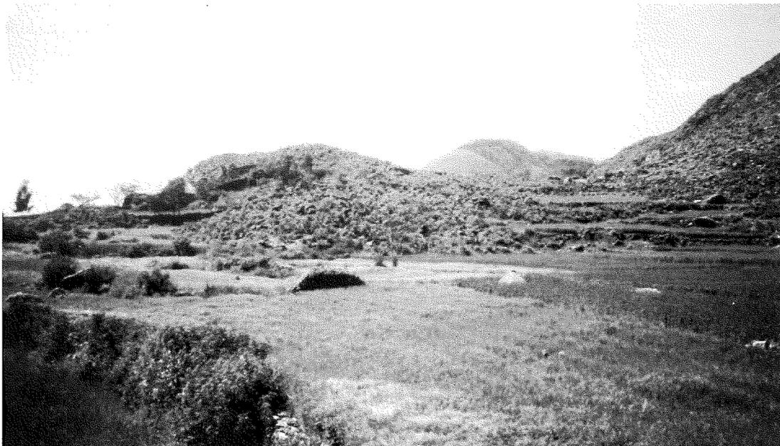
Fig. 3 - Checkdams in a partially filled gully close to Mai Zahla nursery in Dingilet (left: in 1994). In 1997 (right), most of the dams were by-passed or destroyed by floods.
