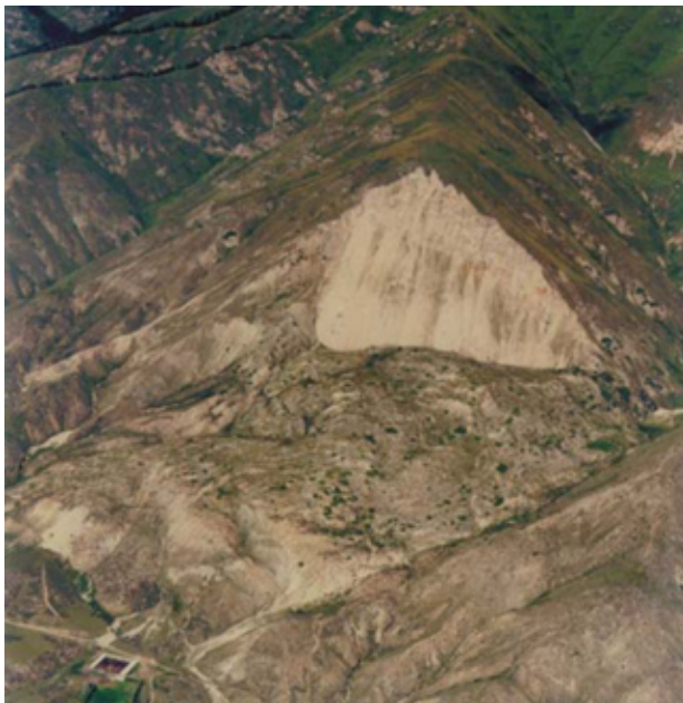
Figure 3: Helicopter Photograph of the Ananevo rockslide ( 10\text{--}15 \times 10^6 \text{ m}^3 ). Scale is given by the horse-farm building (lower left corner) of roughly 60 by 60 m.
