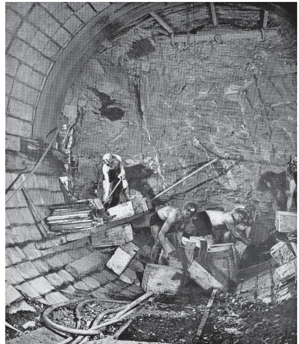
**Figure 5.** Constructing a major gallery in silty claystone rock in the Waterschei colliery (Campine basin), showing decompacted natural fractures and veins (predominantly dipping right with steep angle 67°), besides some rock shattering produced by explosives. Photo Minders, in: Kolenmijnen André Dumont N.V., 1957. Waterschei 1907–1957. Edition L. Cuypers, Brussels (by permission of N.V. Mijnen).
