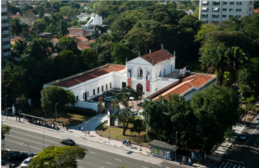
Figure 1 – Aerial photo of the MCB, 10 March 2017.
