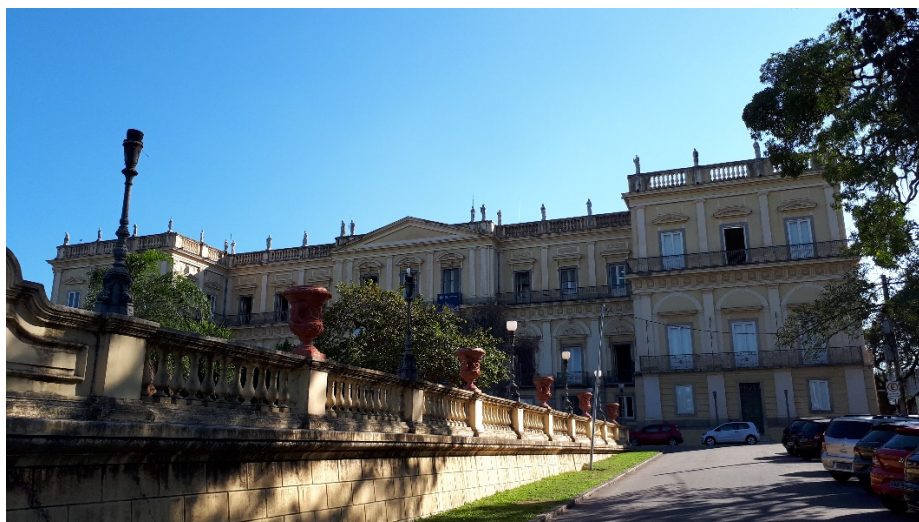
Figure 1 - Main building of the National Museum, four days before the fire.
