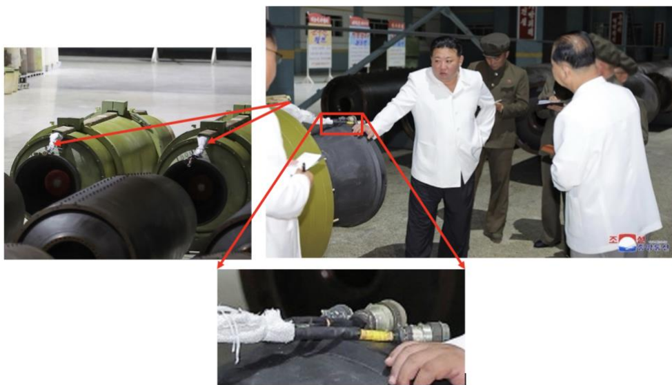
Figure 12. Grey-colored fabric inside and extruding from missile cable ducts seen in photographs inside the February 11 Plant. Source: KCNA image broadcast August 14, 2023.
